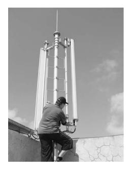
Pic. 5 Operation close to lower edges of antennae
